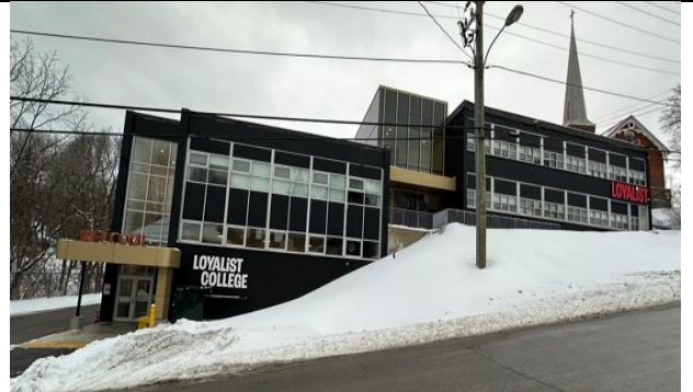
Picture 2. Port Hope Campus 10 Pine Street, Port Hope
